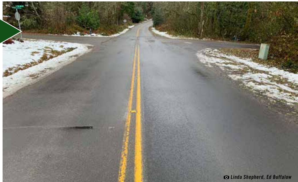
Edge cracking and returning to gravel on 260th Avenue SE at the intersection with SE 157th Street
