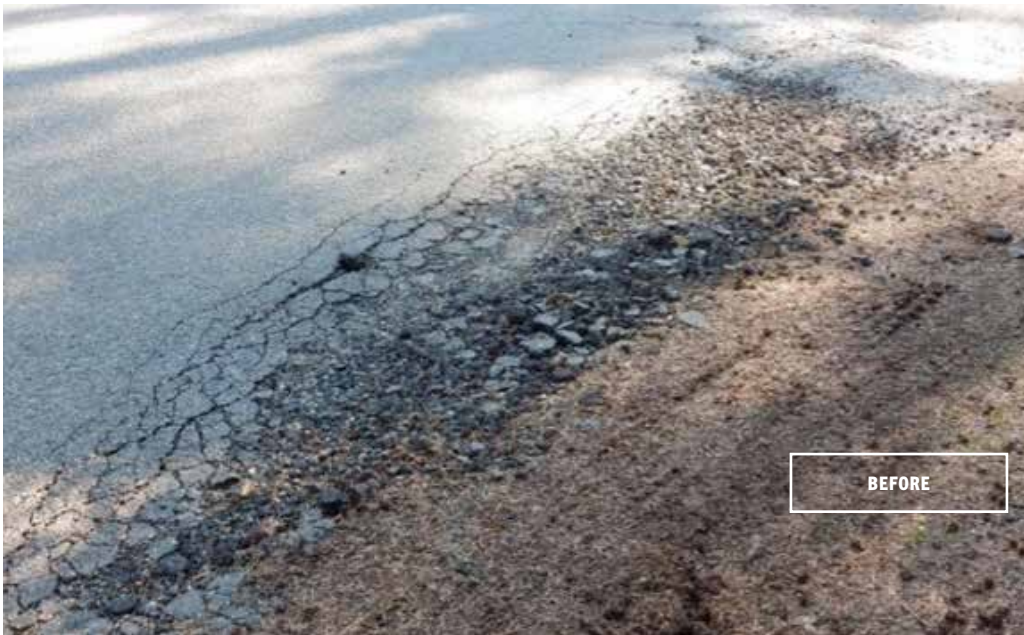
Edge cracking and returning to gravel on 260th Avenue SE at the intersection with SE 157th Street
